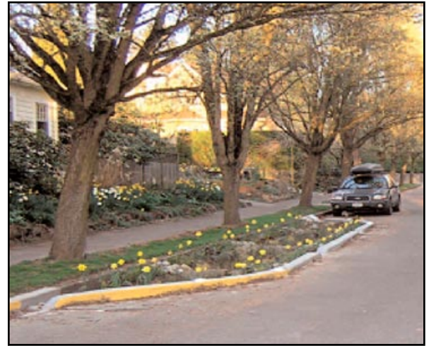
An extended curb design that slows and filters stormwater runoff before it flows into the storm drain. Photo courtesy of Bureau of Environmental Services, Portland, OR
