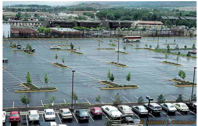
Large parking areas impervious to rainfall, resulting in water runoff.
